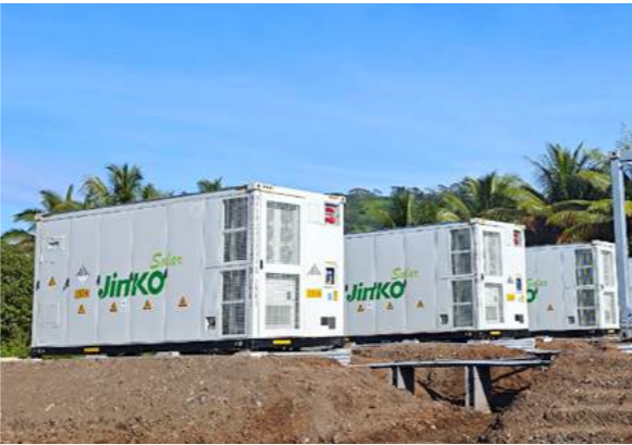
The large-scale solar energy storage project in Tahiti, French Polynesia is equipped with the Blue Whale SunTera energy storage system, which has C5 level corrosion resistance and is suitable for the offshore environmental conditions and climate of Tahiti, ensuring the long-term stability and high durability of the system.
