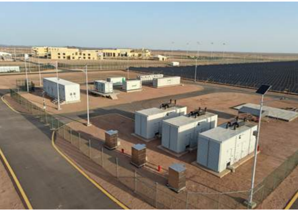
The off-grid DC-coupled cell energy storage system in eastern Saudi Arabia is heat resistant and sand proof, capable of maintaining cell temperatures below 35°C in extreme environments with a temperature difference not exceeding 5°C.
