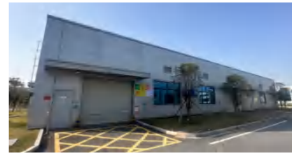
Solid Waste Storage Place
