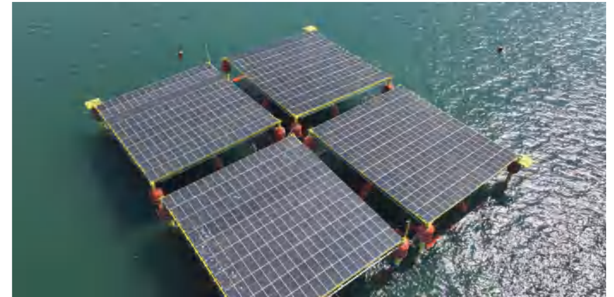
The Company collaborated with CIMC Raffles to develop offshore semi-submersible floating photovoltaic platforms, and explored the weather resistance of floating structures and photovoltaic modules in marine environments and their performance in the face of wind and waves
